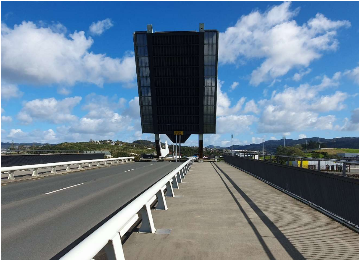
Figure 2-1: TMAP Bascule lifted
