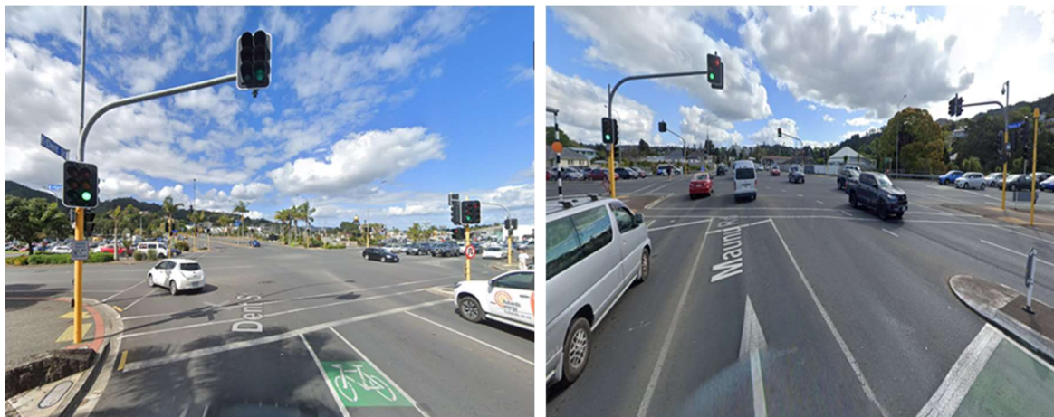
Figure 1-2: Traffic Signal mast arms & lanterns
