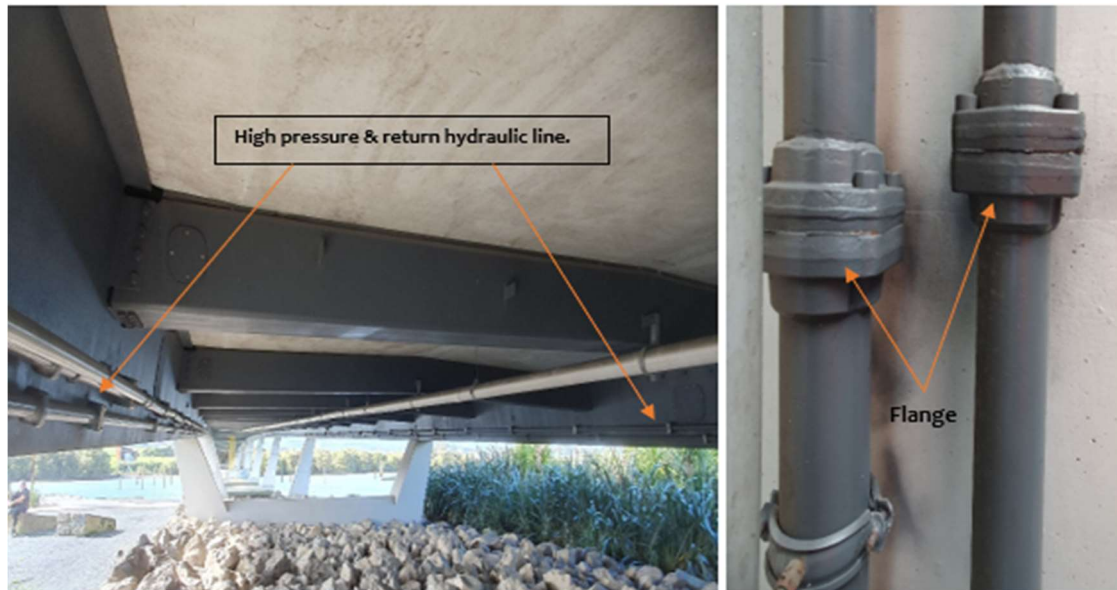
Figure 2-4: Hydraulic pipe network under the bridge
