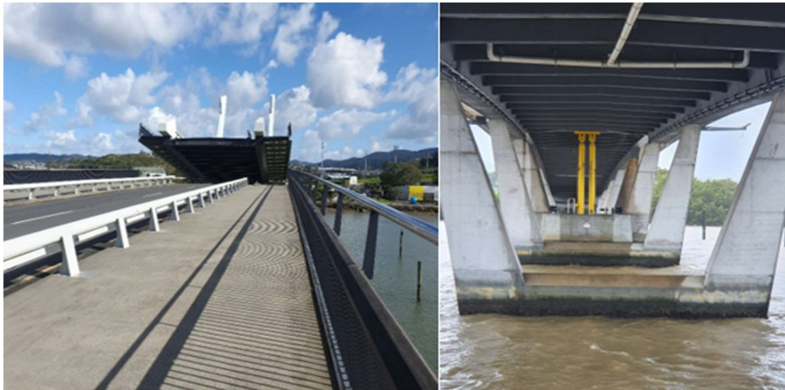
Figure 1-4: - Bascule lifting and Hydraulic RAMs at W1
