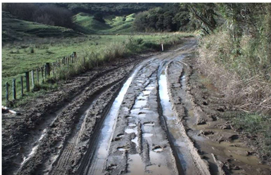
Figure 3-2: Inadequate watertables
