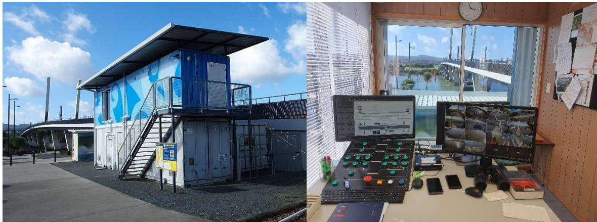
Figure 1-6: Bridge Control Room
