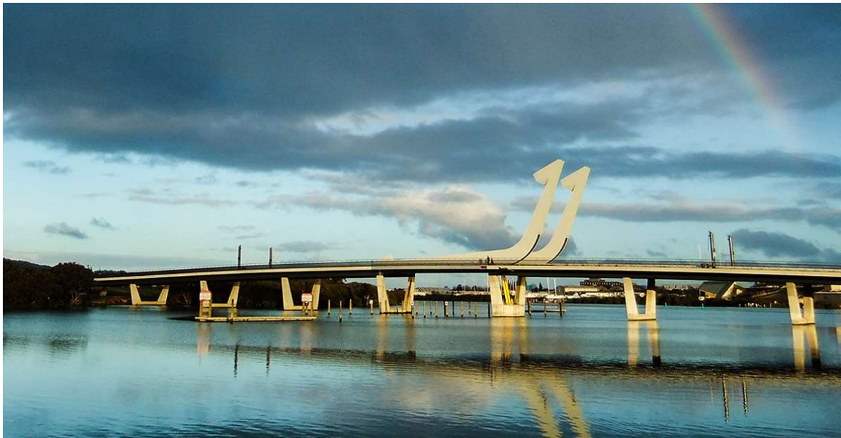
Figure 1-2: Te Matua ā Pohe bridge
