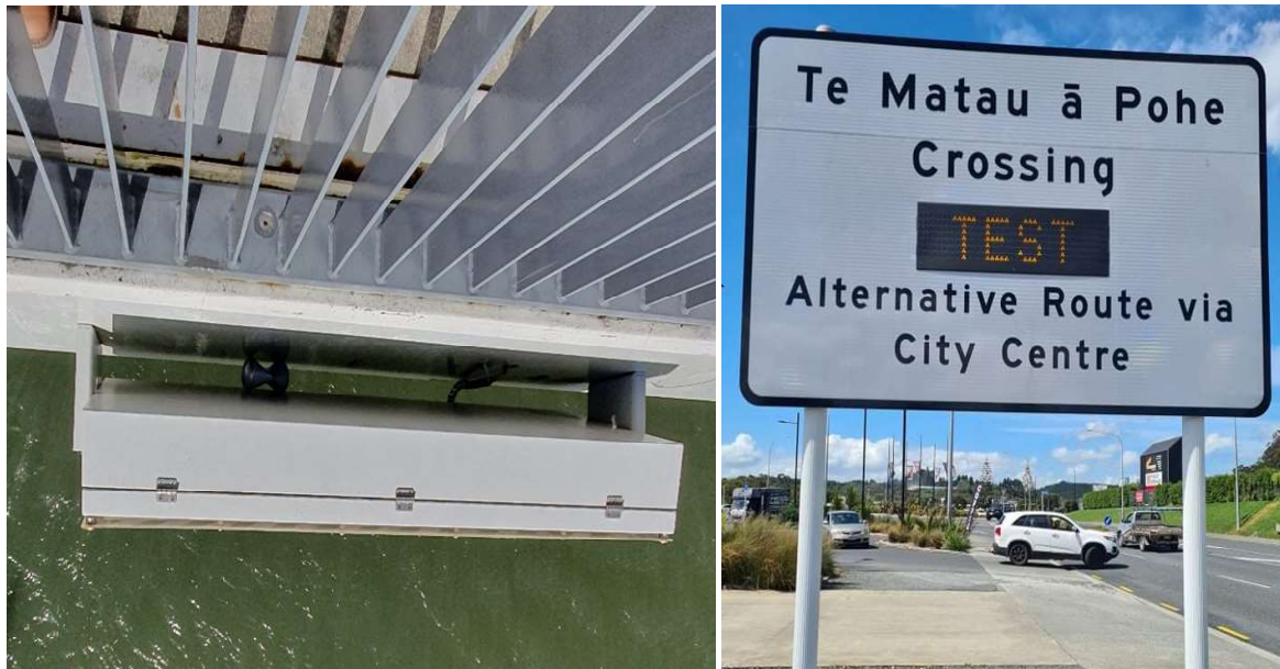
Figure 2-7: Marine VMS to be replaced (LHS) and upgraded road VMS for TMaP bridge (RHS)
