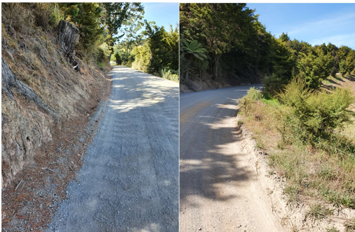
Figure 3-1: Inadequate watertables
