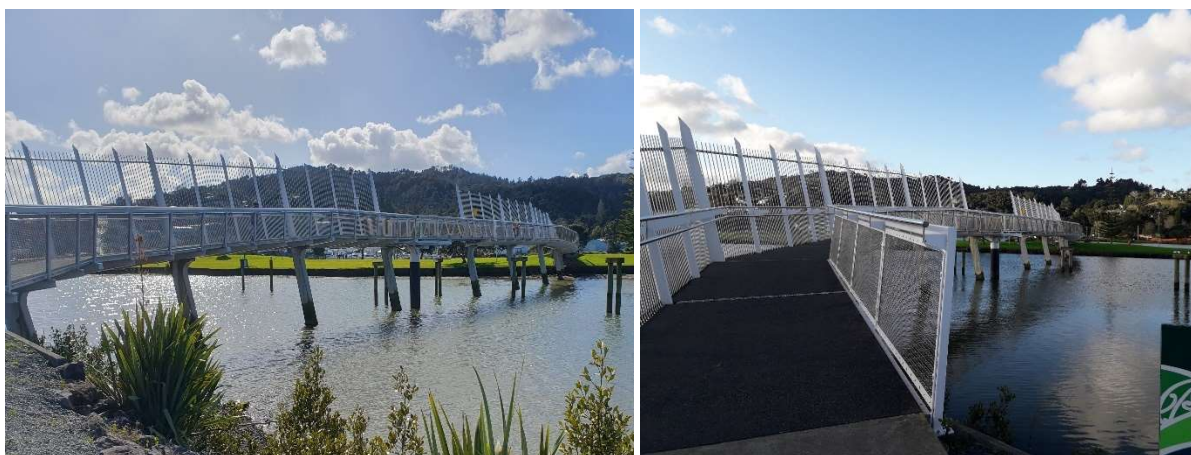
Figure 1-5: Kotuitui Whitinga Pedestrian Bridge
