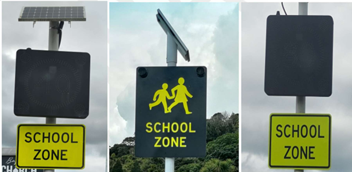
Figure 1-3: Fixed & variable school zone Signs (SZS)
