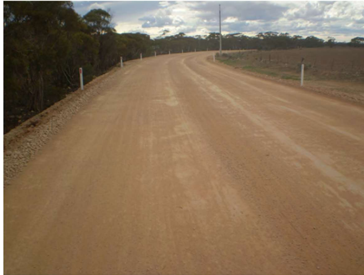
Figure 3-3: Cames Road with Paige-Green compliant
