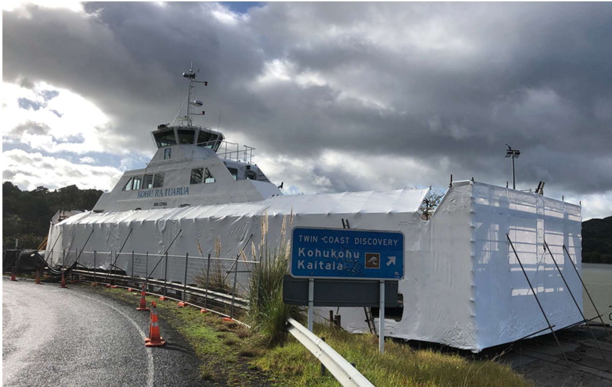
Figure 2-1: Out of water maintenance
