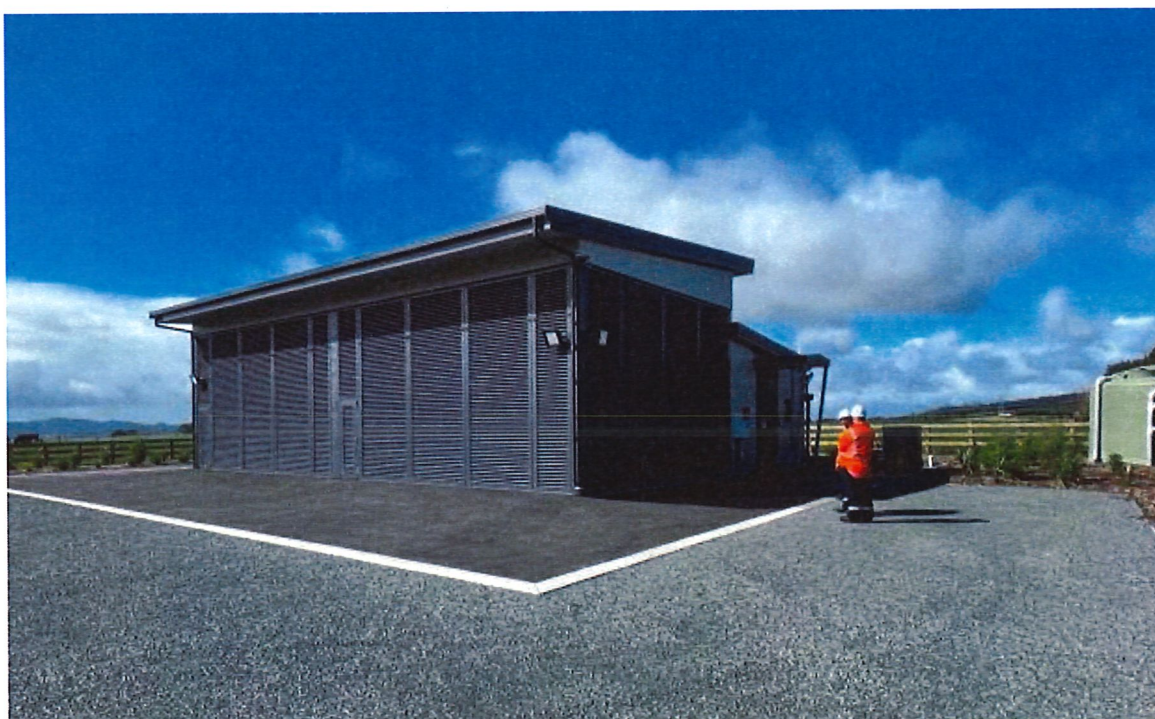
Figure 1: Existing Northpower substation.
